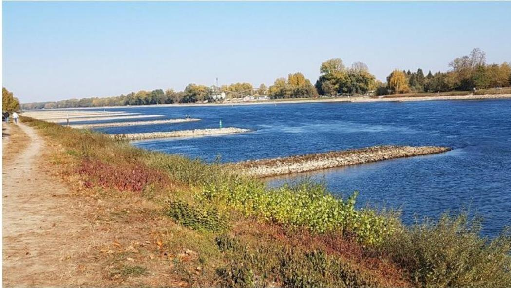
**Figure 33: Groyne system on the shore of the free Rhine part**
