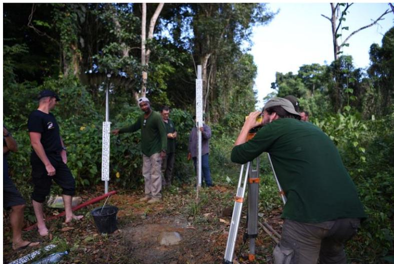
Figure 25: site 2: installation of the gauge at Kio Konde, Tapanahoni river in Suriname
