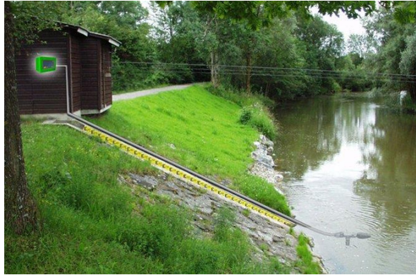
Figure 20: Example of bubbler sensor installed on a river bank
